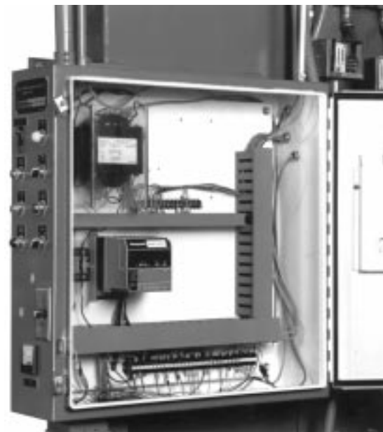
Fig. 11—Electrical panel installation.
