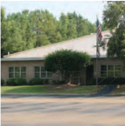
Fluid Control Division Facility, Madison, MS.
